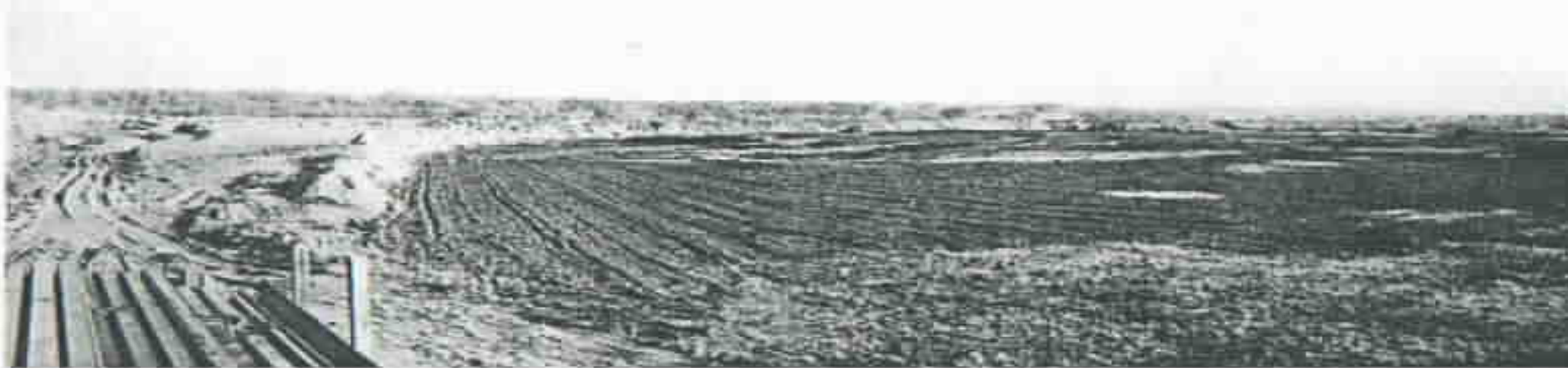
Top soil being removed when yard started.
